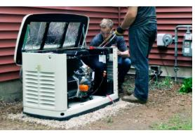
**TIP** When using plantings as a screen to hide a generator, keep the foliage trimmed at least 3 feet from the front and both ends of the box and make sure overhanging branches are at least 5 feet above the top of the box.
